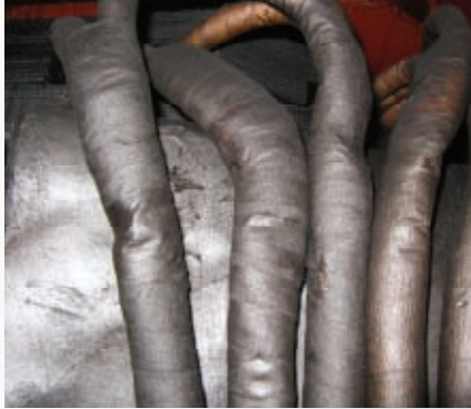
Sludge on the transformer windings
